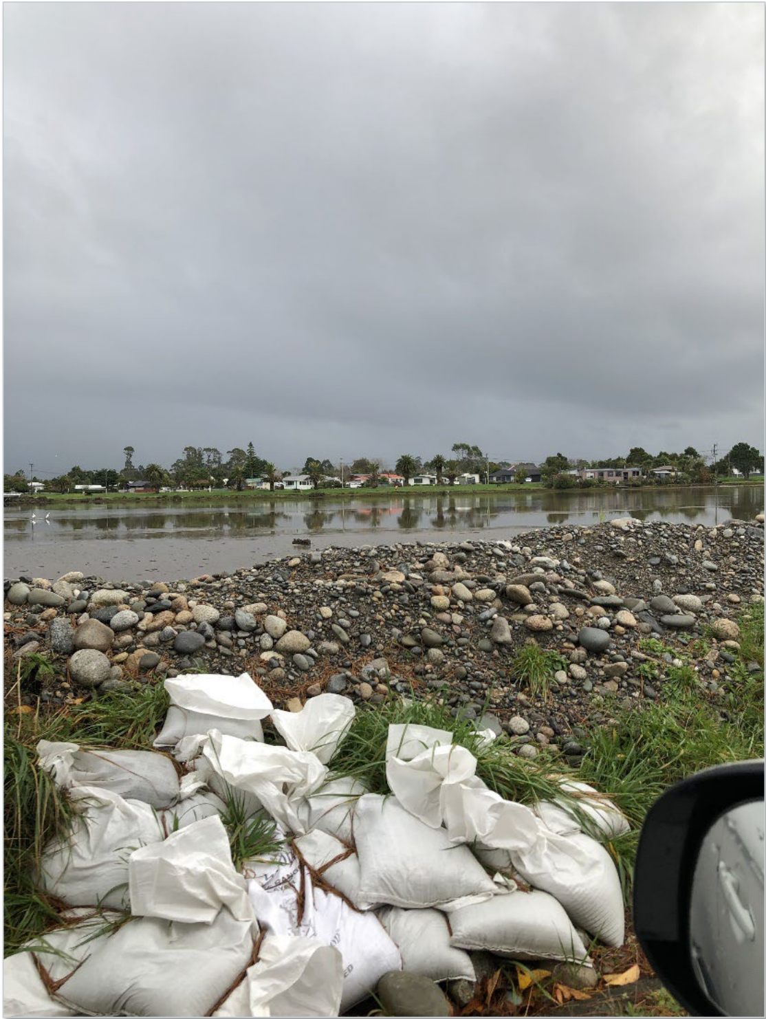
Figure 15 – Temporary stopbank at Snodgrass Road
