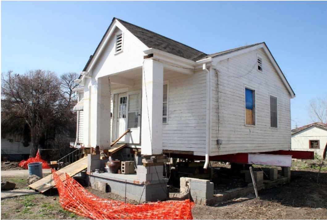
Figure 25 House being raised in New Orleans
