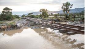
These photos show how flood water escapes once it builds up and flows over the Stephens Road and Railway line abutments.
