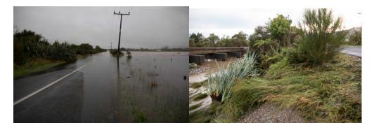
The first photo shows the flood water unable to flow under Stephens Bridge. The second photo shows the height of the bridge abutments against the railway viaduct, restricting the flood water flow.
