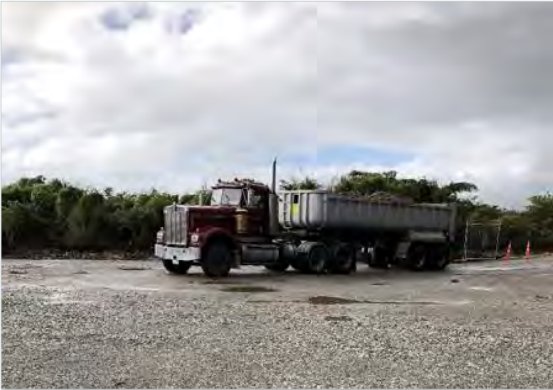
Figure 28 - Earthworks for Temporary Accommodation Service at Alma Rd (photo courtesy Pam Johnston)
