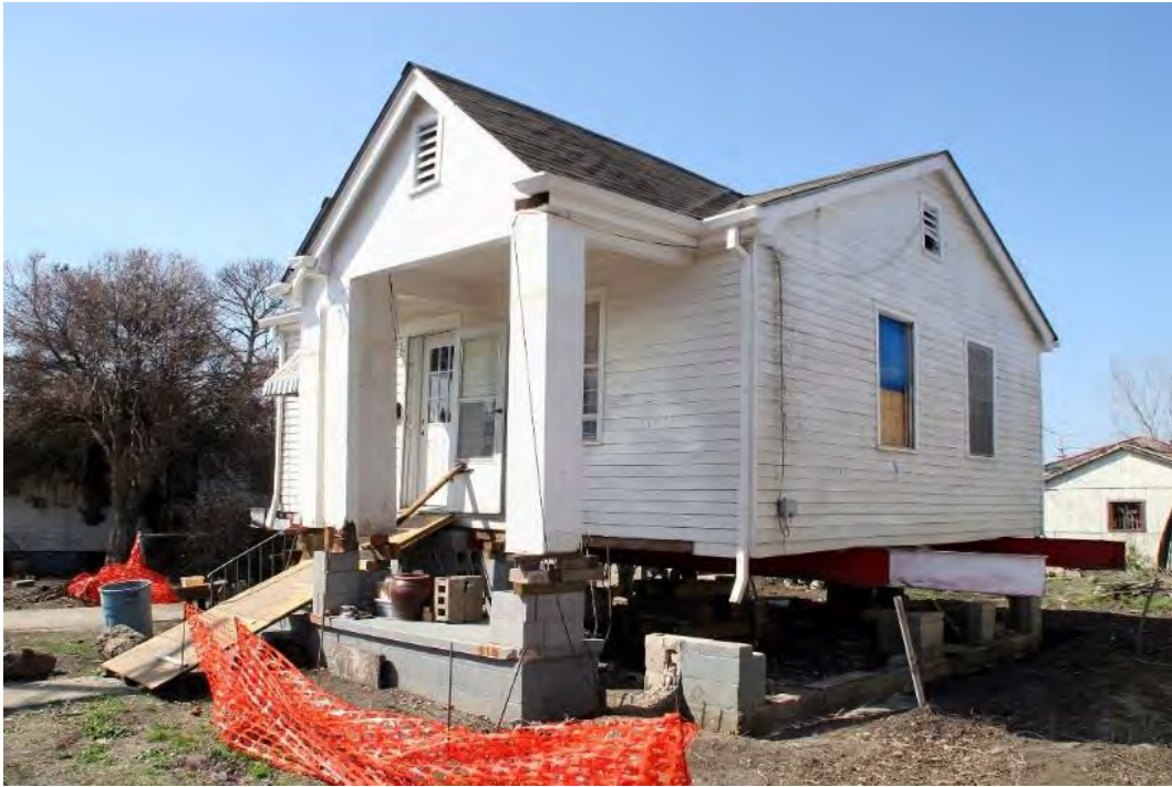
Figure 25 House being raised in New Orleans
