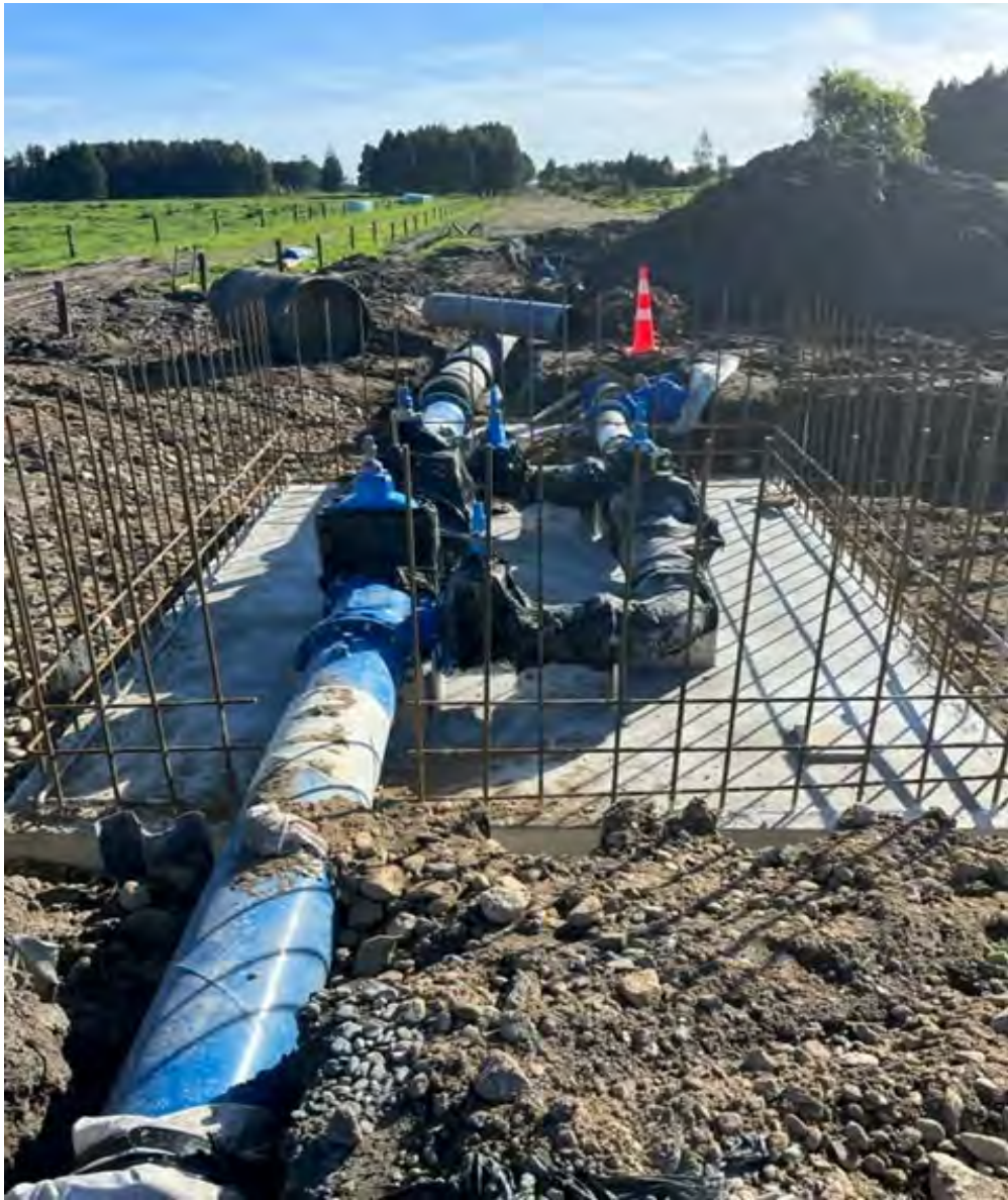
Pressure Reduction Value (PRV) assembly under construction
