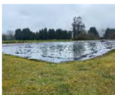
Reefton WWTP Aeration Pond
