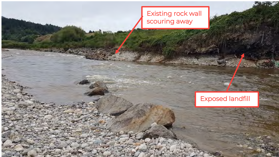
Figure 3. Image of the landfill showing failed rock wall protection
