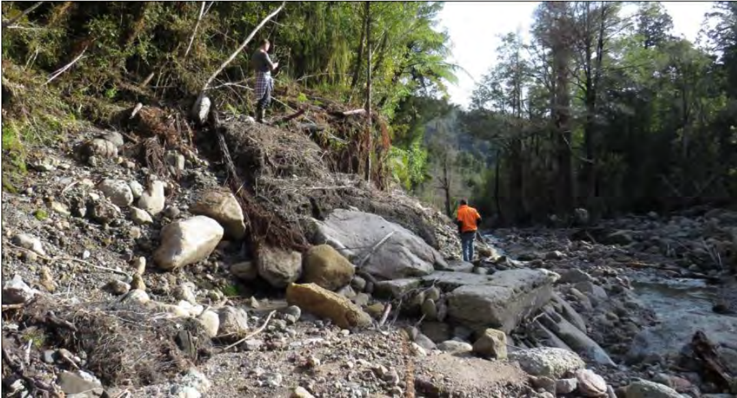
Figure 2.4: Remnant of North Branch historical concrete intake structure destroyed by July 2021 debris flow
