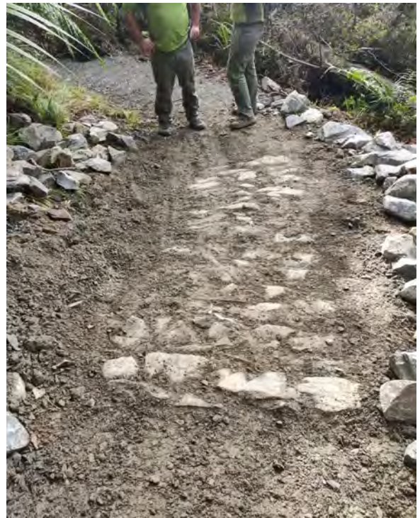
Figure 16. Pitching #2, looking north, soon after completion (left; image: DOC), and as it appeared during the final site survey (right).
