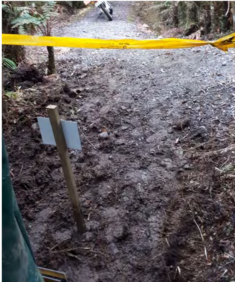
Figure 13. Junction 7, looking west along the existing track, following excavation. There does not appear to be any original track fabric visible. Image: DOC.
