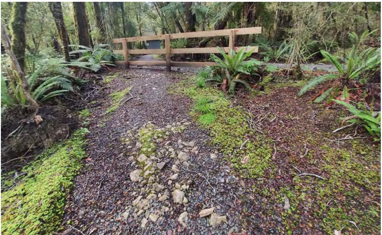
Figure 6. Junction #4 as it appeared during the final site survey. This photo taken from roughly the same position as Figure 5, showing the original track running from the foreground towards the top of the image and the new track section on the right. Note, the original track basecourse material in the foreground has been largely unaffected by the work.
