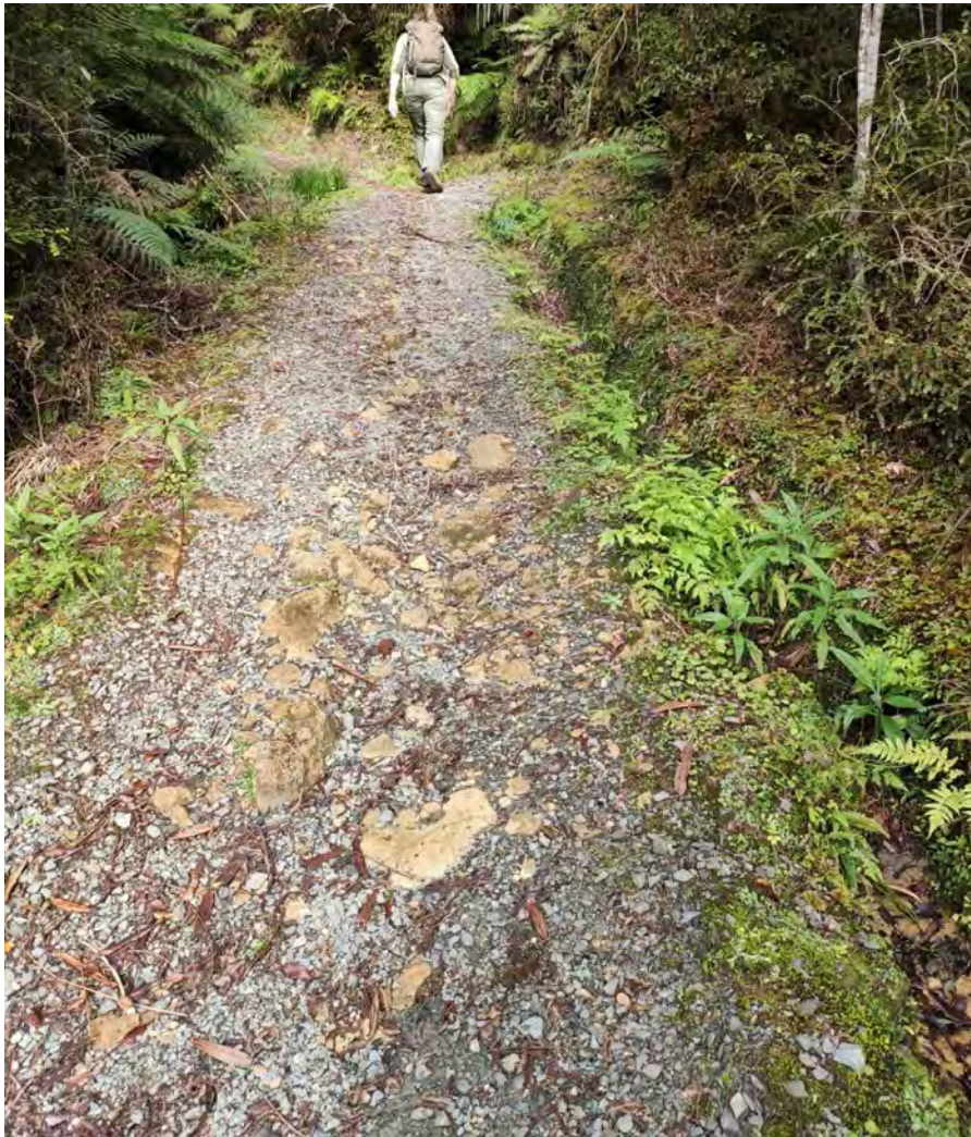
Figure 21. A section of the track between Junctions 4 and 5 with original base course and side drain that was unaffected by the project.
