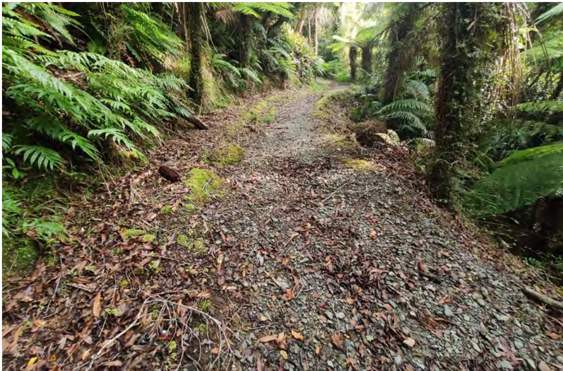
Figure 22. A 1/2 benched section of the track that was unaffected by the project.
