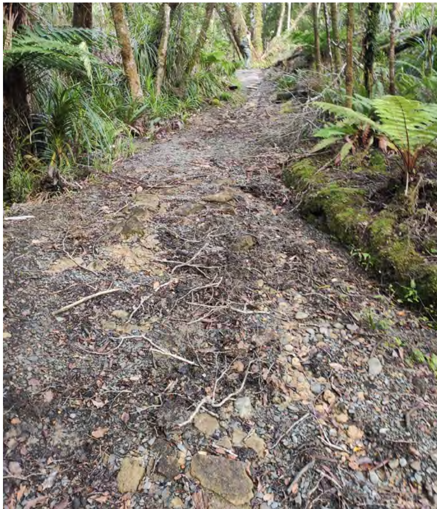
Figure 20. Track surface damage between Junctions 4 and 5, this section is likely water damaged also.
