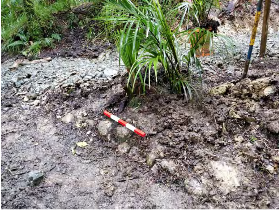
Figure 11. Junction #6 after the new surface was added to the new section. The original track edge, indicated by the scale, was not affected. The base course for the new track has been placed behind the nikau. Scale: 500 mm, 100 mm increments.
