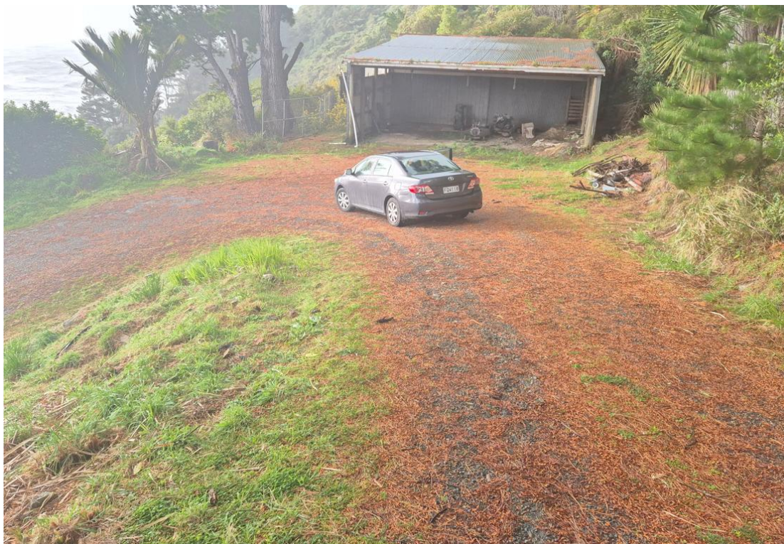
Figure 10. View of the existing shed located near the site entrance at Perpendicular Point (Te Miko). The photograph looks northward, showing the gravelled forecourt and surrounding vegetation.
