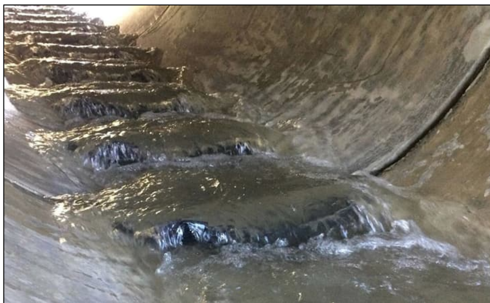
Plate 2: Multiple Flexi-Baffles are placed in a culvert to alter the flow while providing rest areas for species travelling upstream. (Source: https://www.ats-environmental.com/solutions/culvert-baffles/ )
