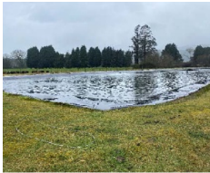
Reefton WWTP Aeration Pond
