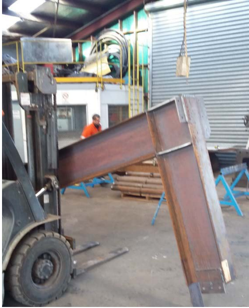
Portal steel corner beam to post; fabrication in the factory.
