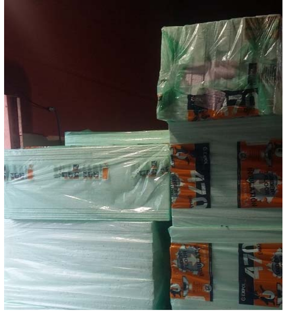
Theatre underfloor insulation prior to installation.
