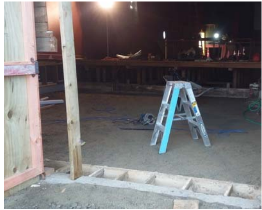
Theatre Storeroom – Preparation of floor slab prior to reinforced concrete pour.
