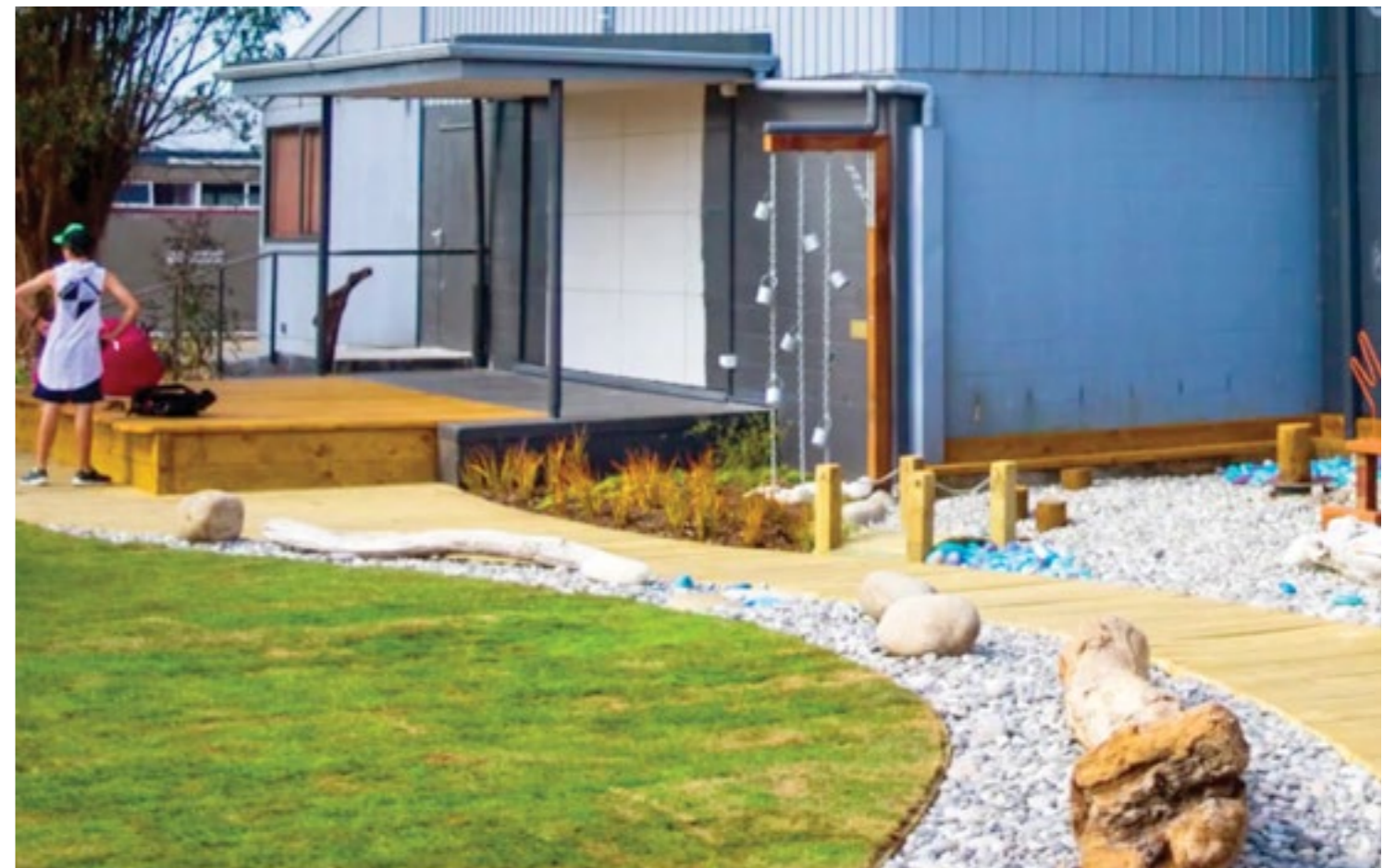
NBS THEATRE ENTRANCE & PARK - AFTER
