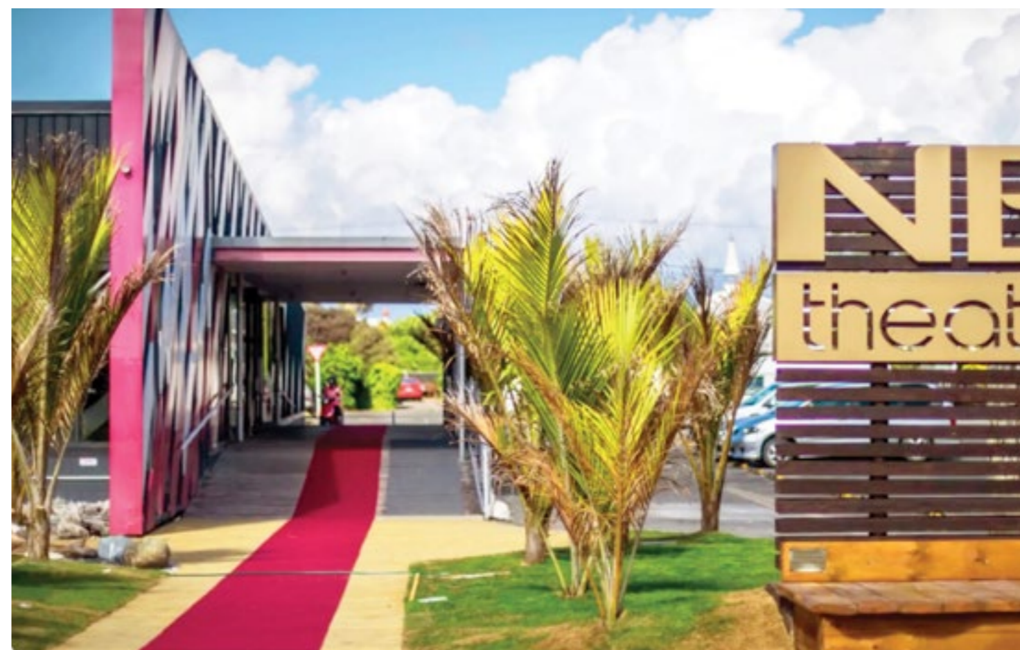
NBS THEATRE ENTRANCE & PARK - AFTER
