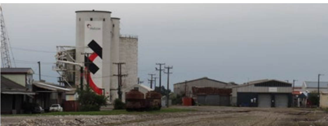
POORLY DEFINED SPACE AROUND THE RAILWAY LAND
